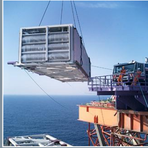
Maintenance, modifications and operations
